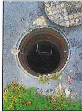
Photo 28: Sewer manhole (typical)
