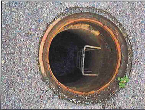
Photo 27: Sewer manhole (typical)
