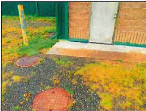
Photo 15: Manholes outside WTP
