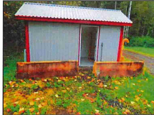
Photo 20: Hagwilget water supply building
