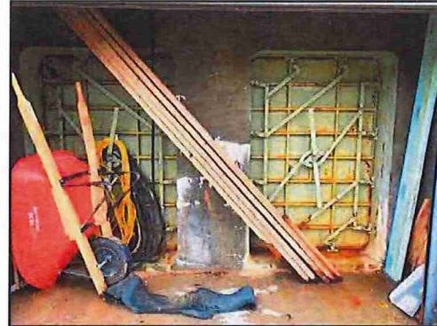
Photo 12: Sand filter access
