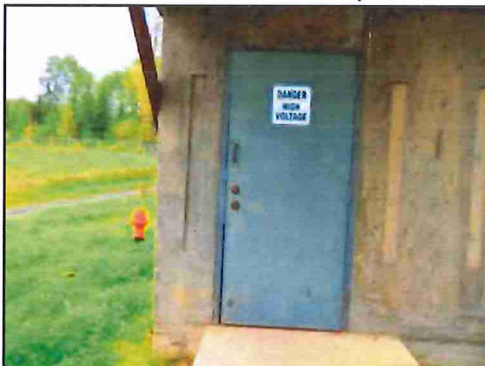
Photo 9: Old water treatment plant
